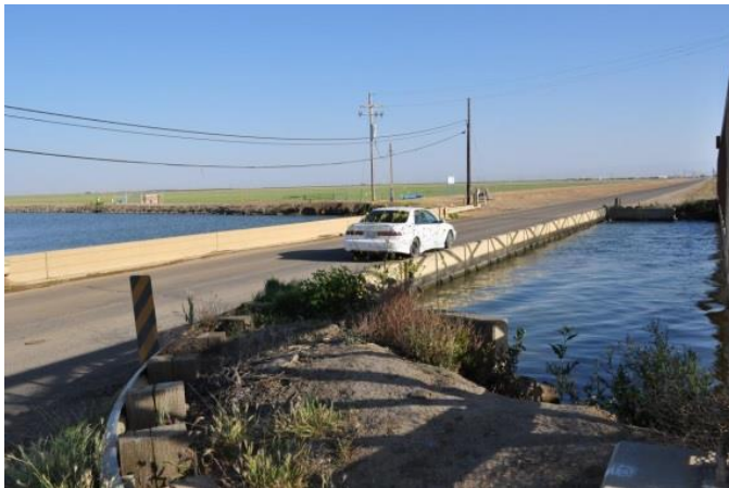
Fig. 5 The submerged Russell Avenue bridge over the Outside Canal, in north of Mendota, California [5]
