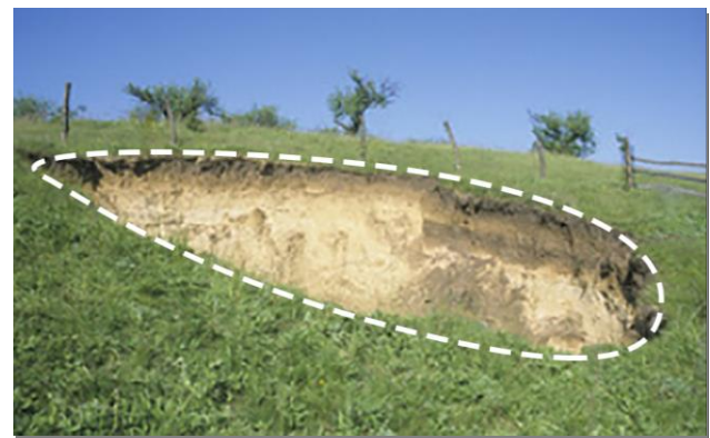
Fig. 8 Danvisky Cover-Collapse Sinkhole; appeared on January 1998, western Ukraine. Adapted from [1]
